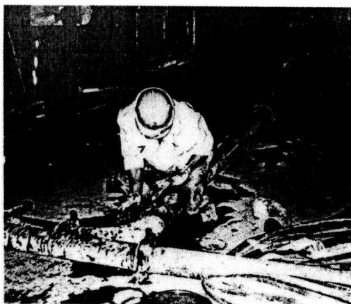
Figure 6 Set up pumping pipe
