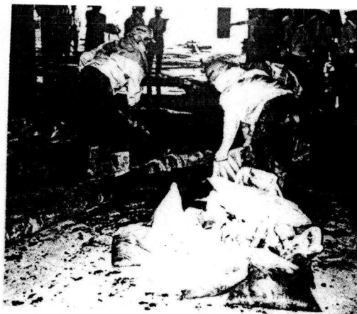
Figure 7 Clear up spilled concrete
